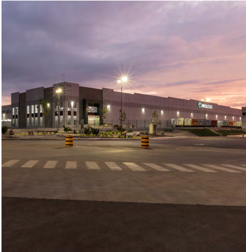
Park Grande, Building 1, Mexico
