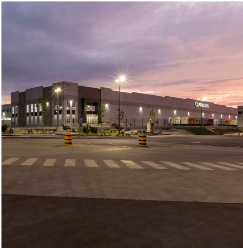
Park Grande, Building 1, México
